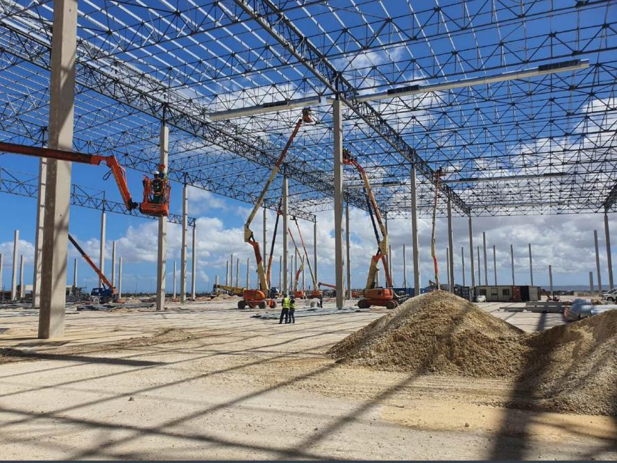
Stability is achieved by designing the columns as cantilevers with moments transferred into foundations
