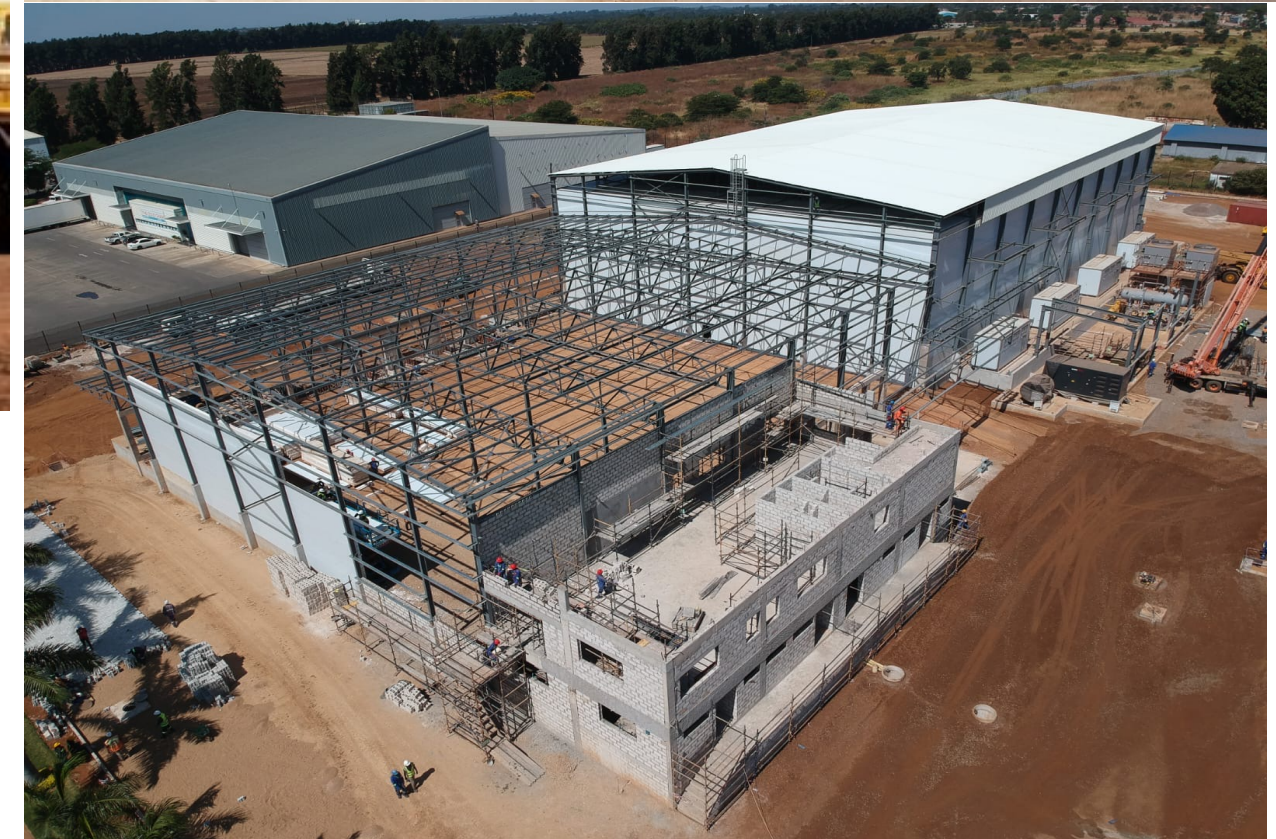
LUSAKA COMMERCIAL COLD STORE
