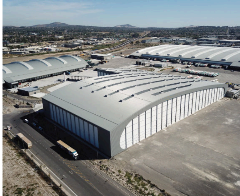
Shoprite Cilmor distribution centre
